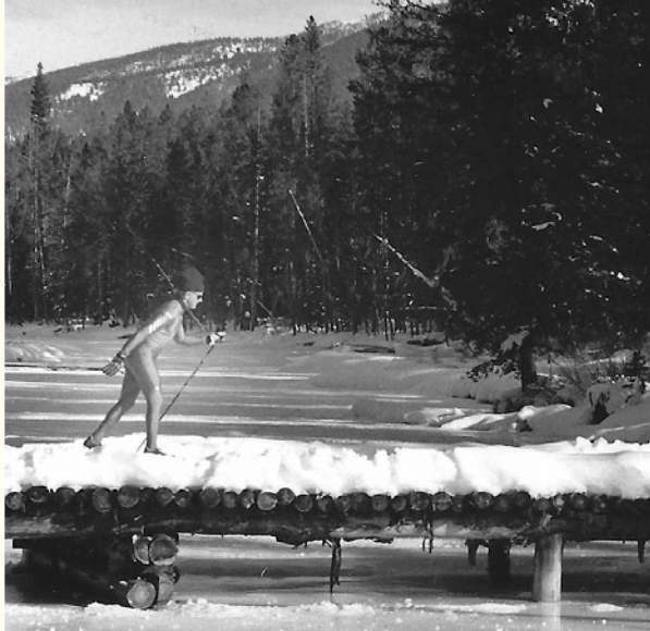
A skier crosses the temporary bridge in 1985.
